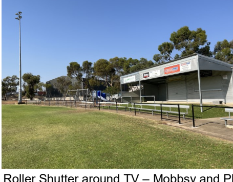
Roller Shutter around TV – Mobbsy and Plumbs
